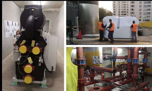
A technical heat recovery system will redirect the released energy by the BCE data centre to heat the RTL city building.
